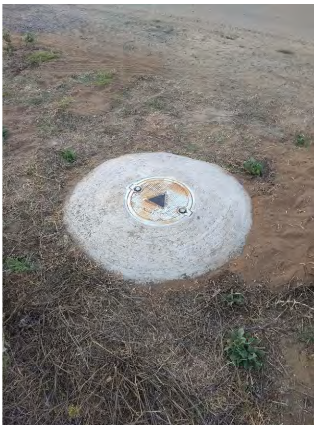
Figure 1. Typical 12-inch monitoring well box
